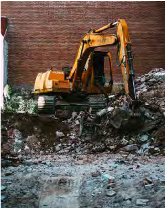
Figure 22.1. A history of construction activity at an urban site oftentimes results in compacted soil that contains both debris and contaminants. Photo by Francisco Andreotti.
