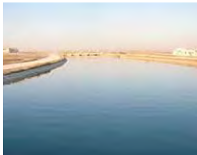
Figure 17.2. The Ataturk Dam, part of the GAP project in Turkey, diverts water from the Euphrates River (left). The main canal (middle) conveys water to the Harran Plain for distribution to individual fields (right).
